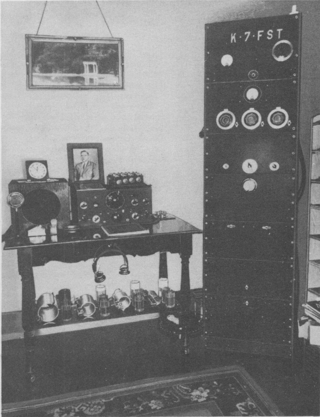
K7FST hits the jack pot with this prize-winning station. Tube line-up in the r-f section is 6L6 oscillator, 802 doubler, 807 buffer, and 2-808's final. Audio section ends up with a pair of 838's. Says K7FST, "I have always been a 100% RCA Tube user. They give you the biggest value ever." Thanks, Om.
